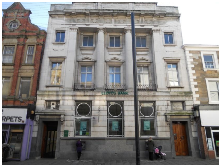
Existing Image: 101 King Street
